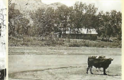
Elkhorn Ranch was located 35 miles north of Medora. Today only foundation blocks mark the site of this second home.
